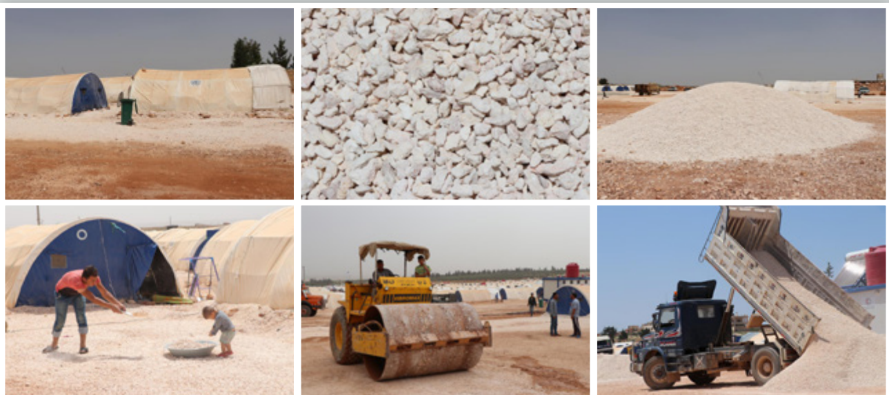
Drainage stones to prevent water inflow into the tents and for general cleanliness of the ground
