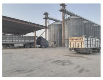
After the quality check the harvest is dropped into an pit underneath the ground from where it is moved into the big Silos by electronic suction control.
